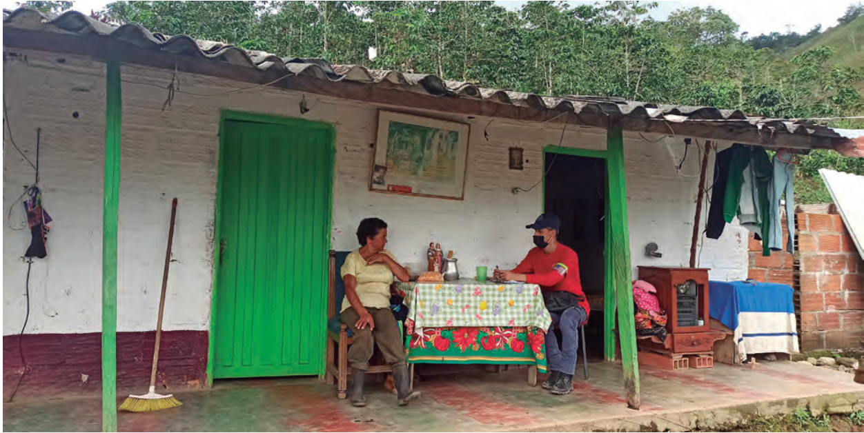
An example of a typical house in rural southern Antioquia.
